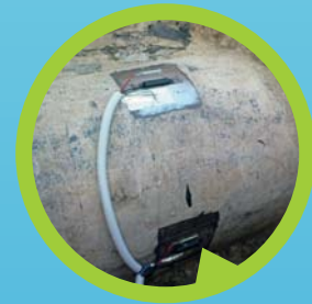
gas pipeline (Posádka pri Hlohovci) placed 10 meters under the ground
